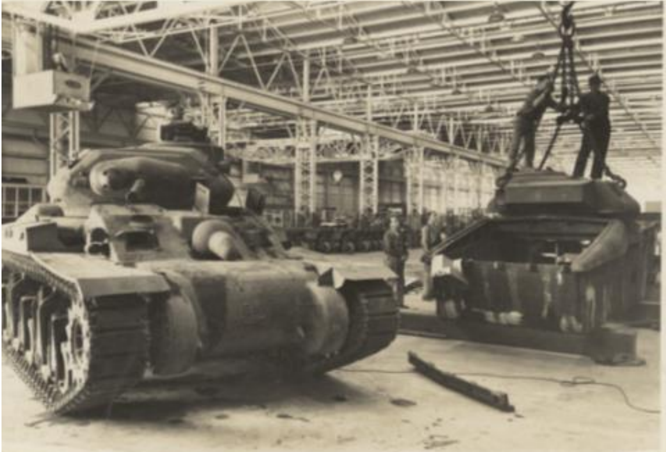
CHULLORA ANNEXE - ANOTHER VIEW OF ASSEMBLY BAY. 25-9-42
